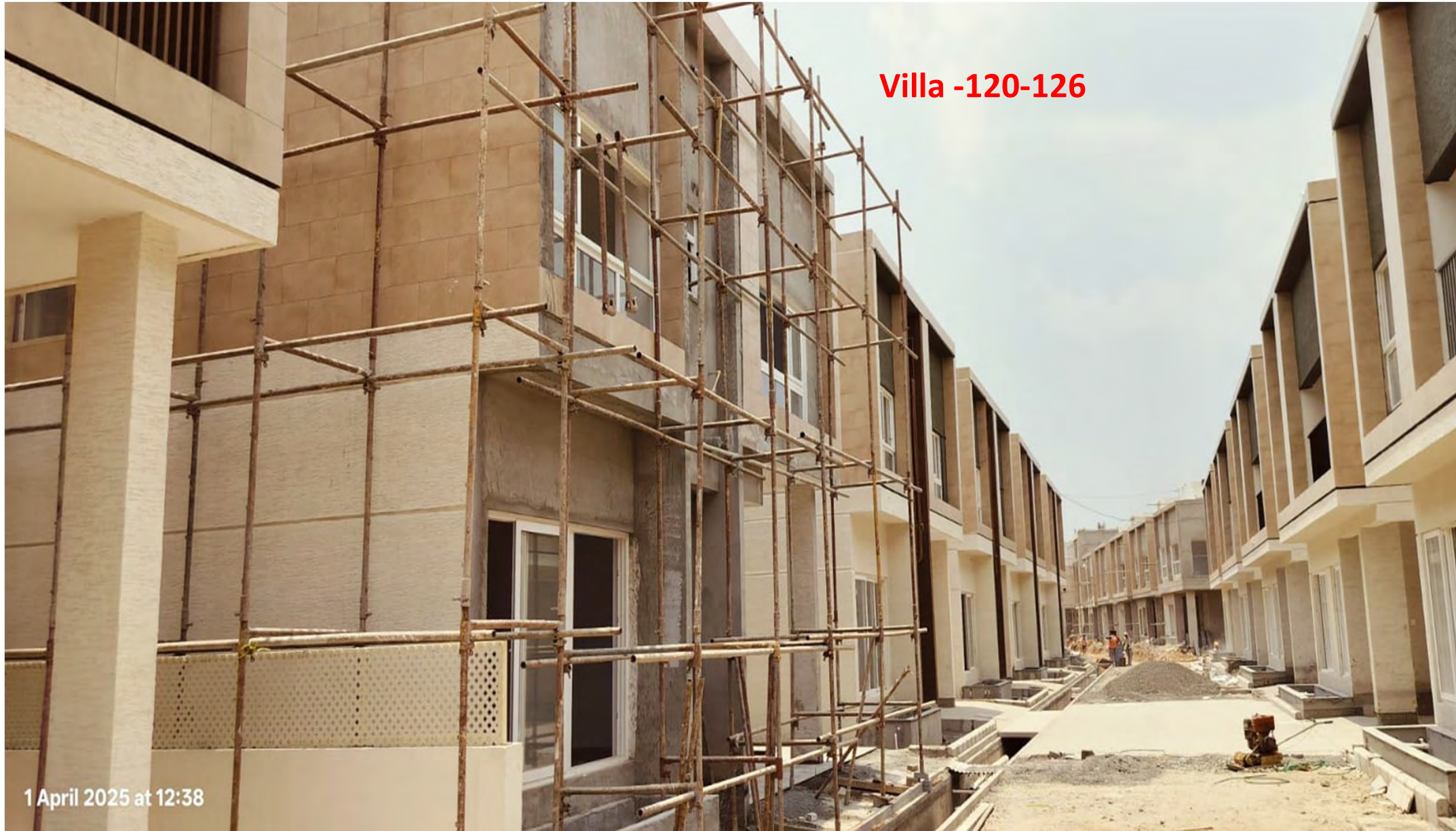
VILLA No's 120-126 Outer grouting work & road sample paver in progress
