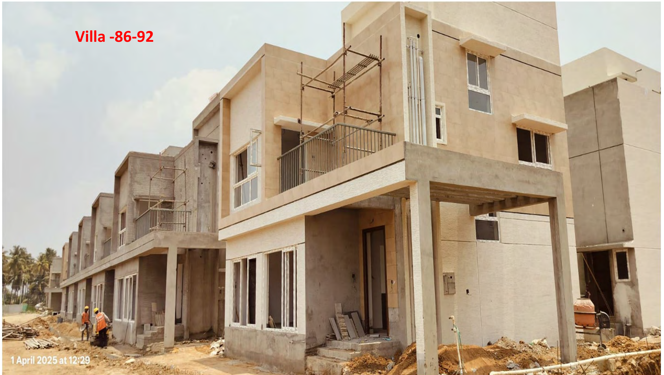
VILLA No's 86-92 outer tiles work in progress
