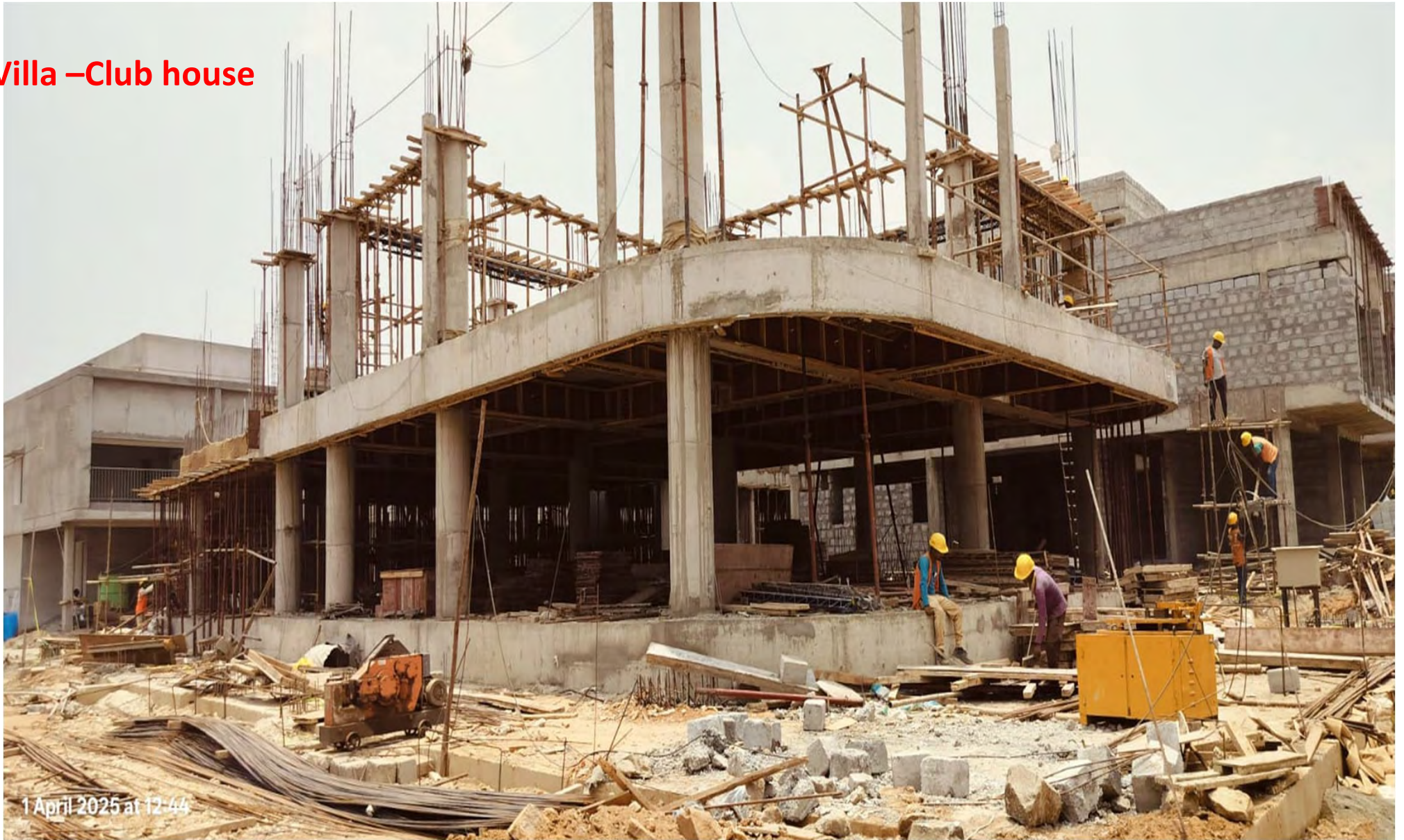
Club house 1 st floor Roof beam bottom shuttering in progress
