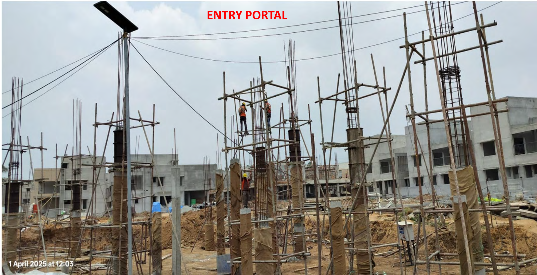
Entrance portal GF Columns Reinforcement-2 nd Lift in progress.
