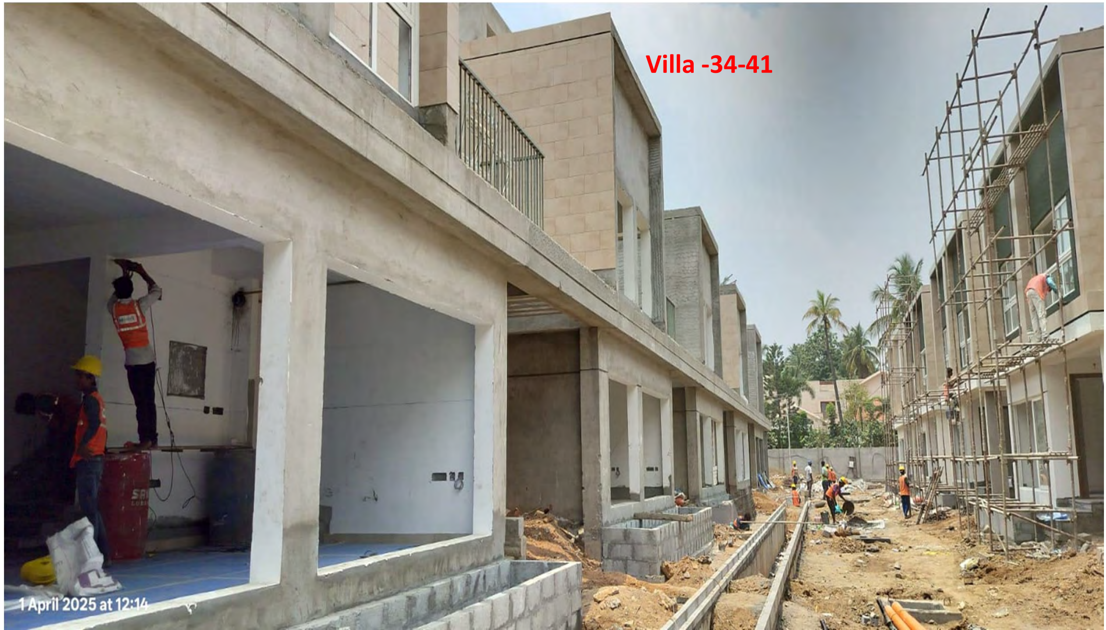
VILLA No's: 34-41 Ready for outer painting & Road Trench work in progress
