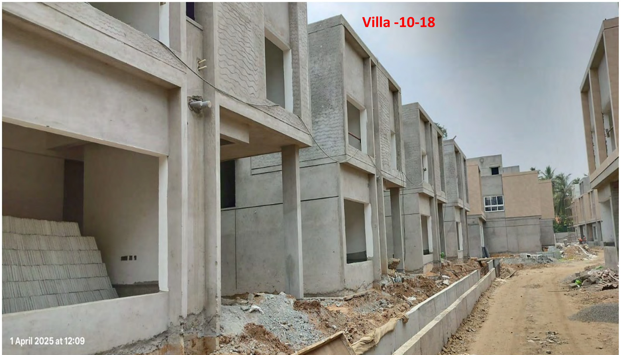
VILLA No's: 10-18 inner & outer tiles work in Progress
