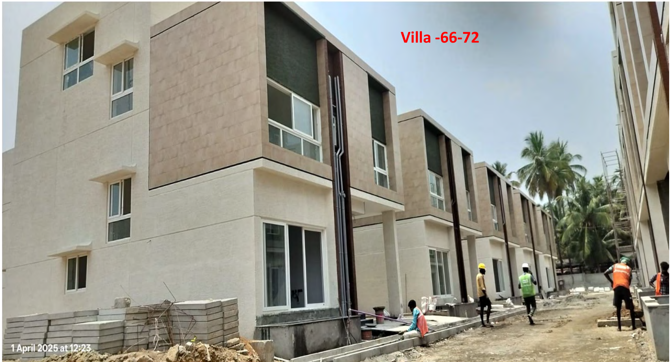
VILLA No's: 66-72 Car parking tiles work in progress
