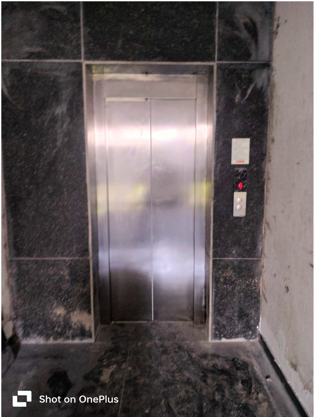
Lobby Flooring & Lift Work
