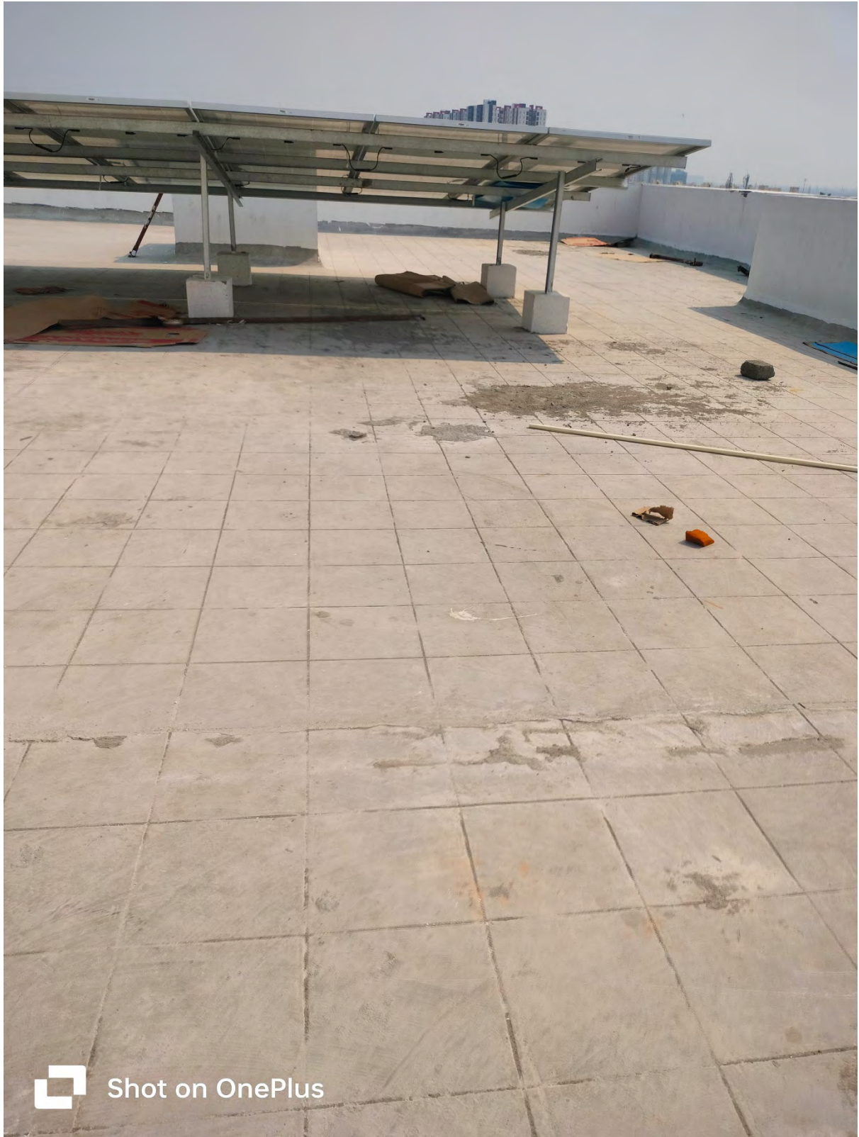
Terrace Flooring Work
