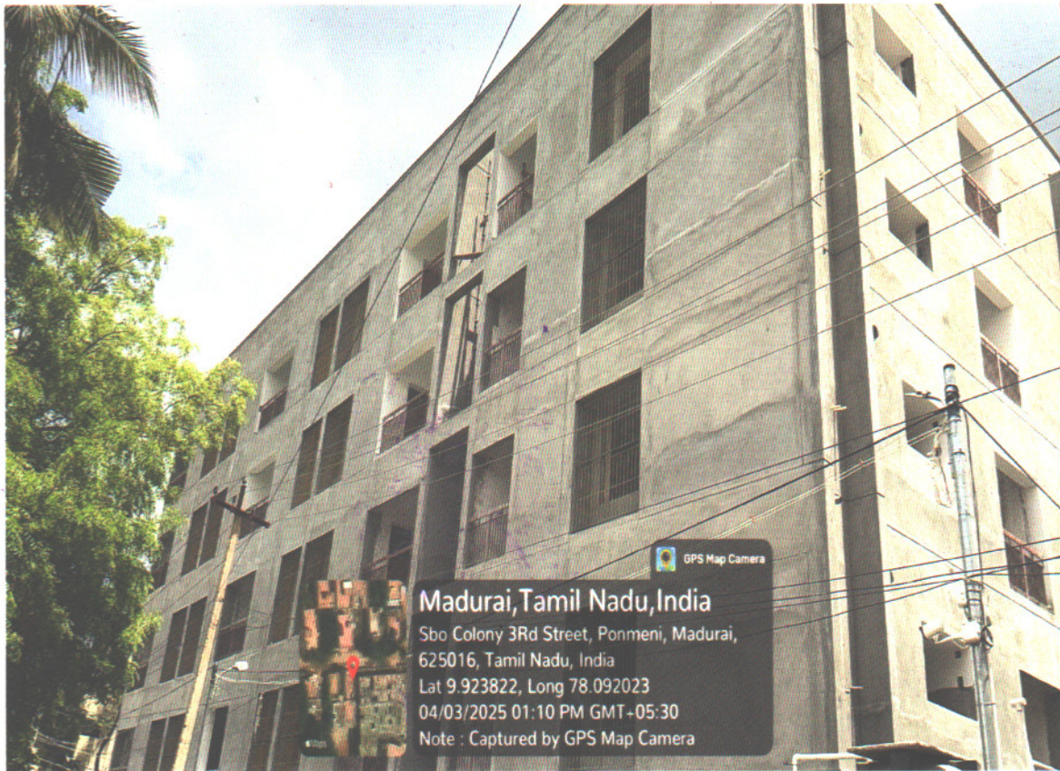
Figure 1 Plastering Under Progress Flooring Under Progress
