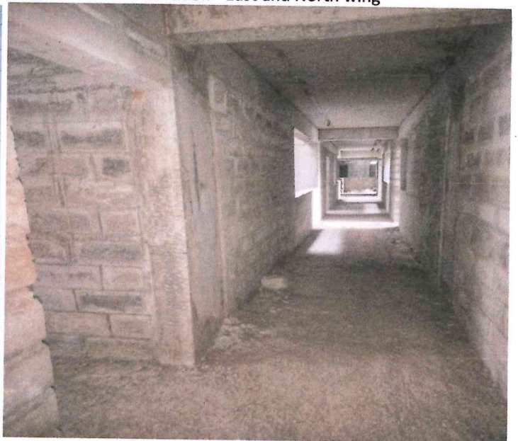
Block work completed – first and second floor
