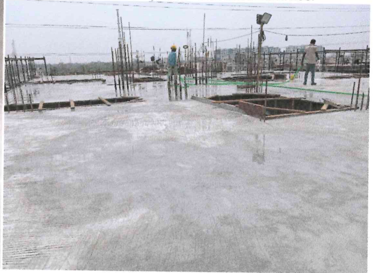
Terrace floor concreting work
