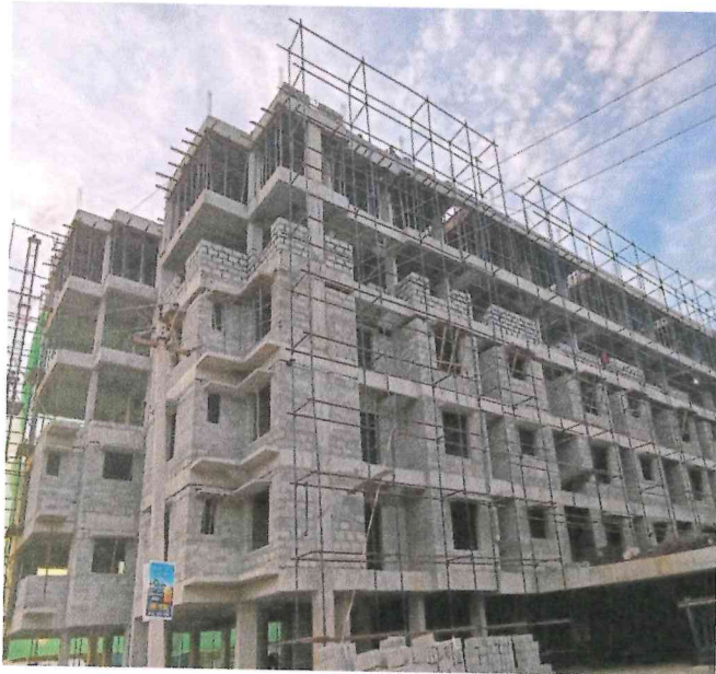
Blockwork in progress in third and fourth floor
