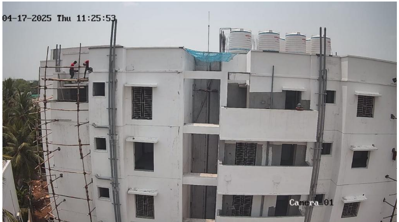
WEST SIDE VIEW
