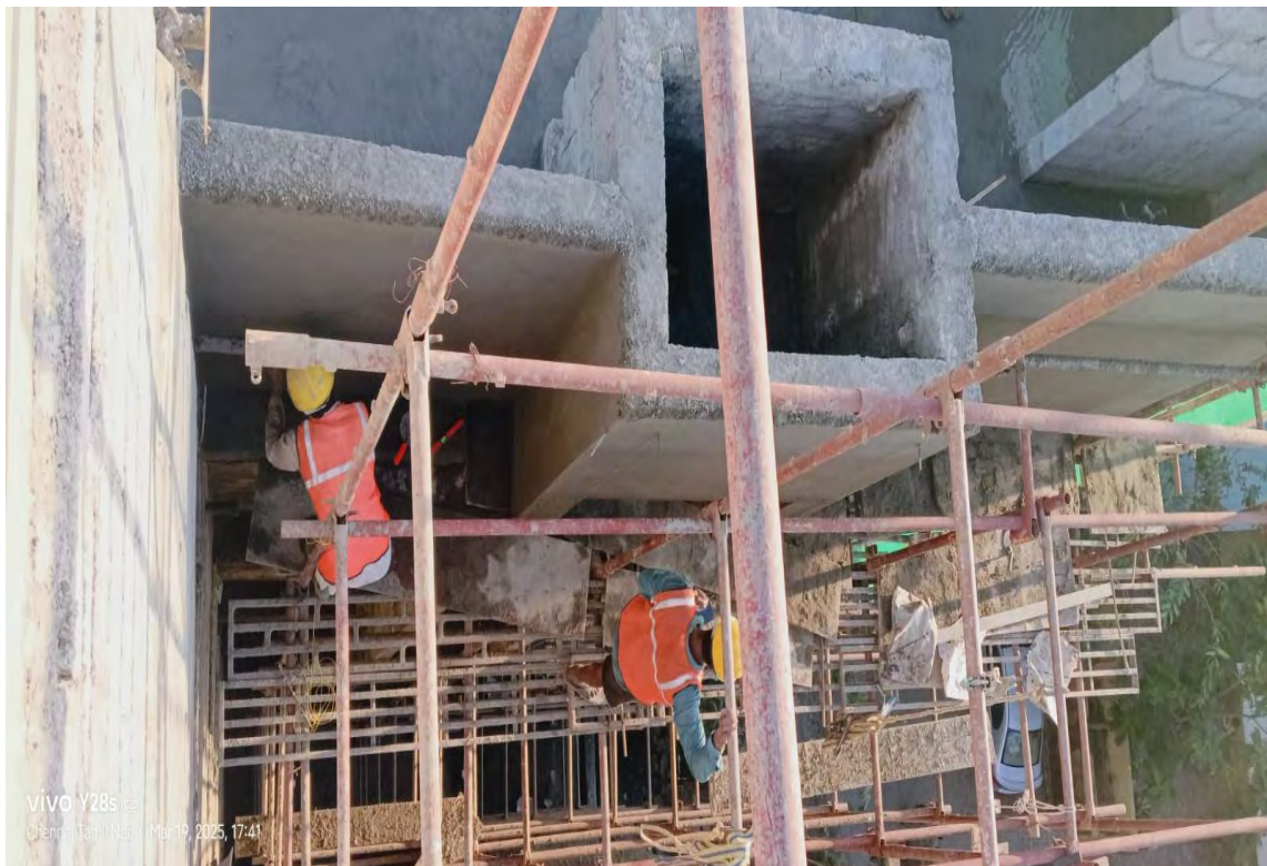
West side OTS 2nd Coat Plastering Works
