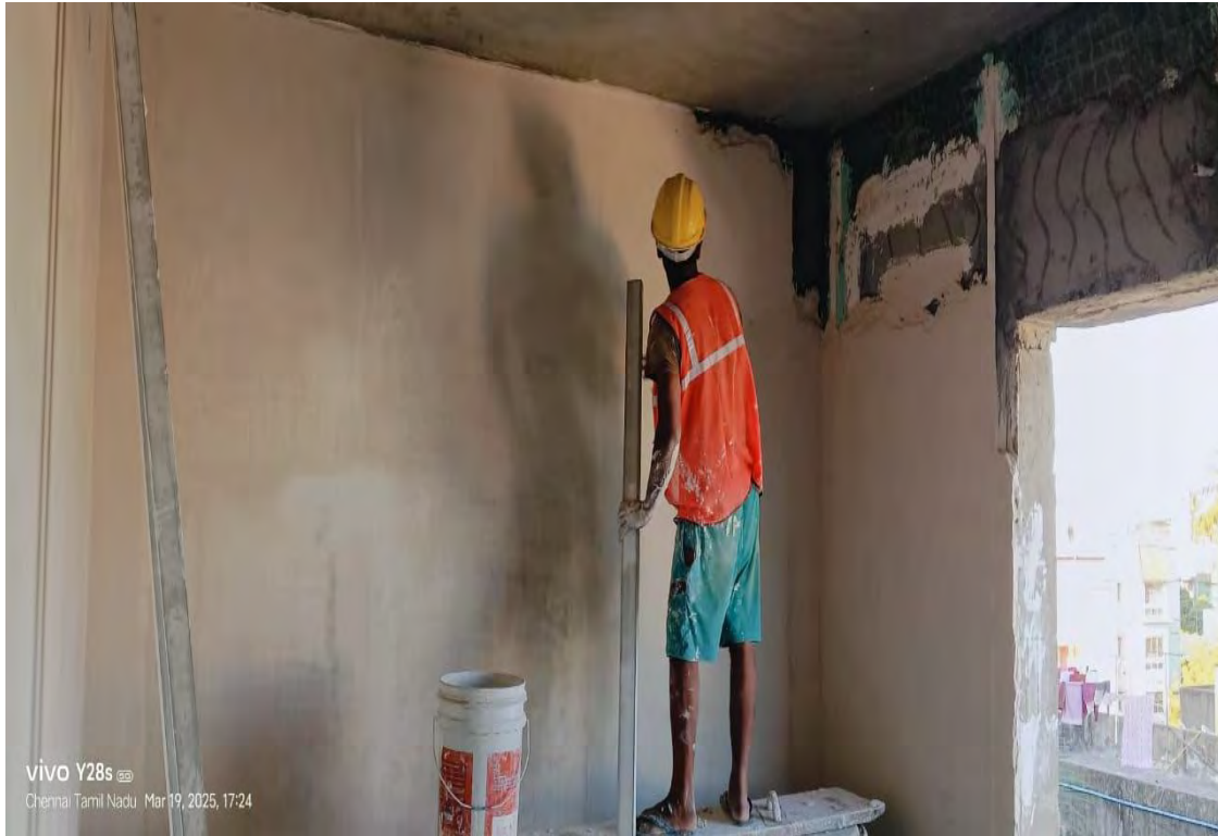
Gypsum Plastering Works.
