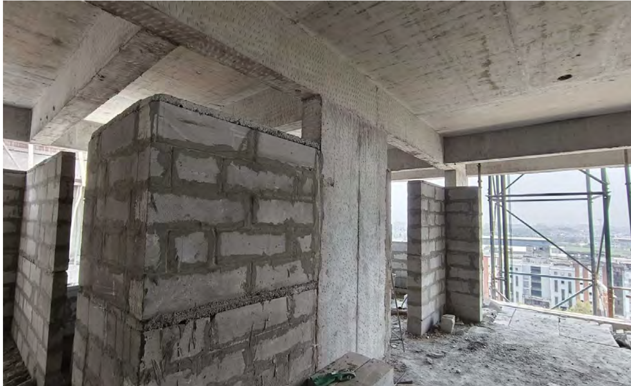
BLOCK 1 - THIRTEENTH FLOOR BLOCK WORK IN PROGRESS
