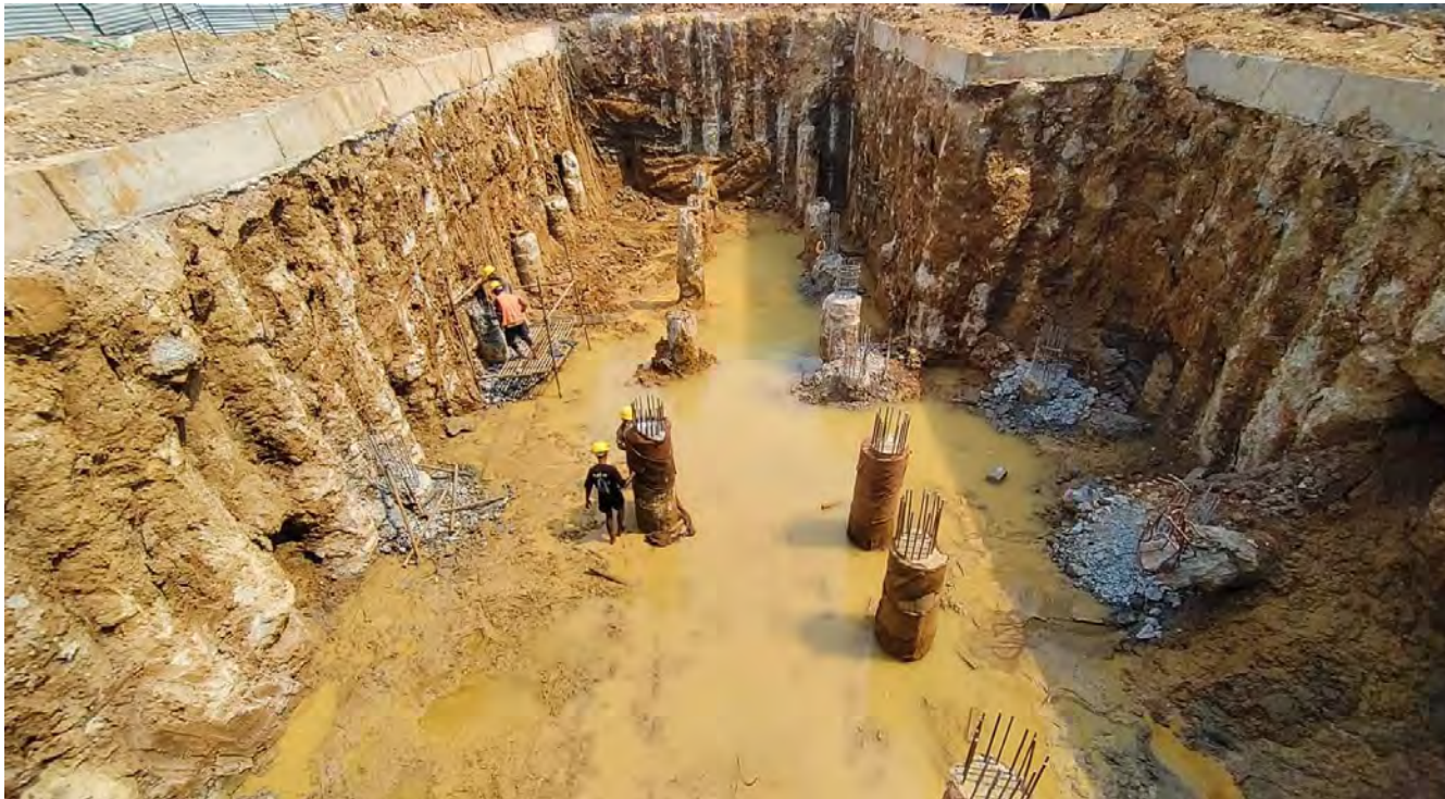
STP - PILE GROWING WORK IN PROGRESS
