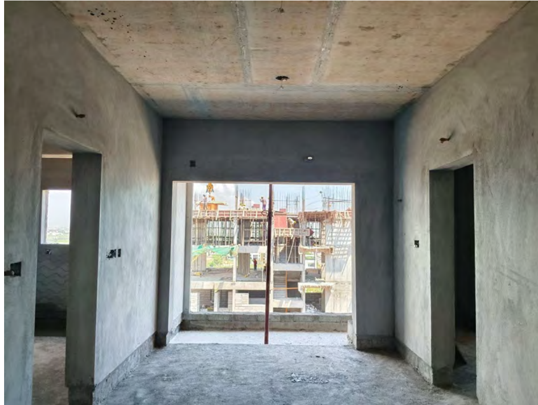
BLOCK 1 - ELEVENTH FLOOR INTERNAL PLASTERING WORK COMPLETED
