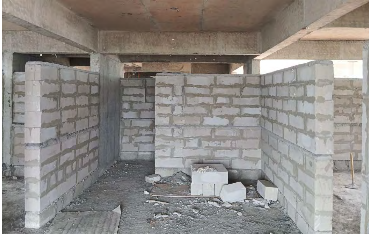
BLOCK 2 POUR 1 - TENTH FLOOR BLOCK WORK IN PROGRESS
