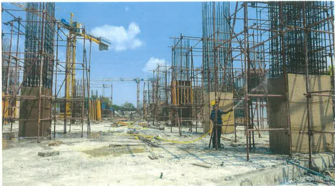
GROUND FLOOR - Column Reinforcement & Shuttering Work In progress
