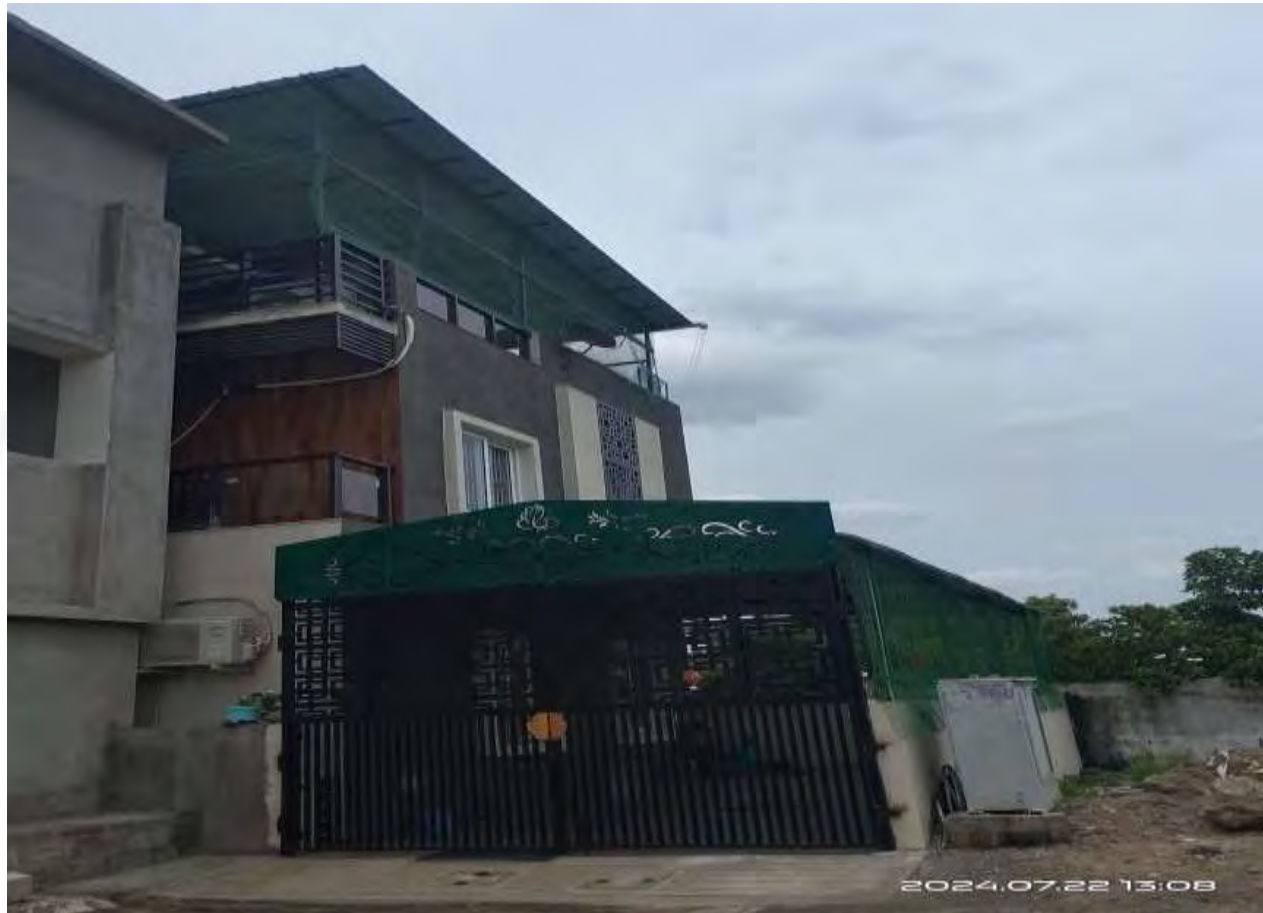
Villa 4 – 100% work completed
