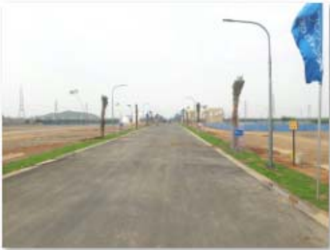
Road work completed
