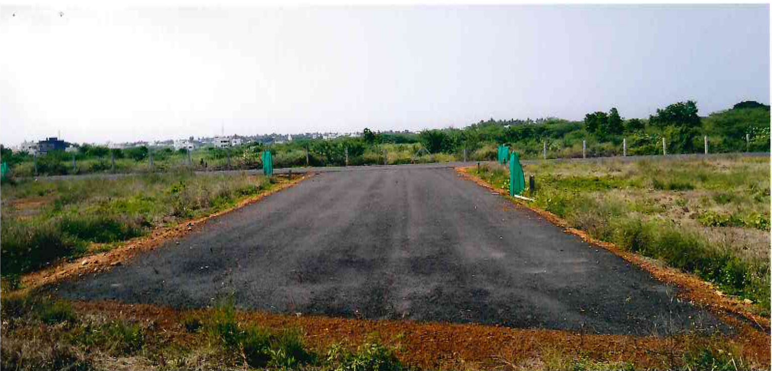
E Boundary - W Facing Road 2-2
