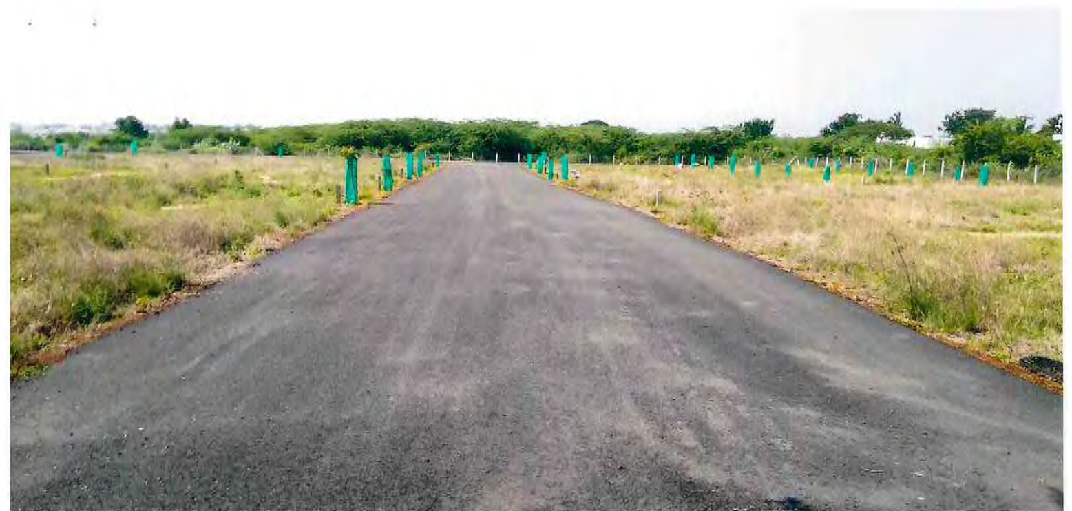
E Boundary - W Facing Road 4-4
