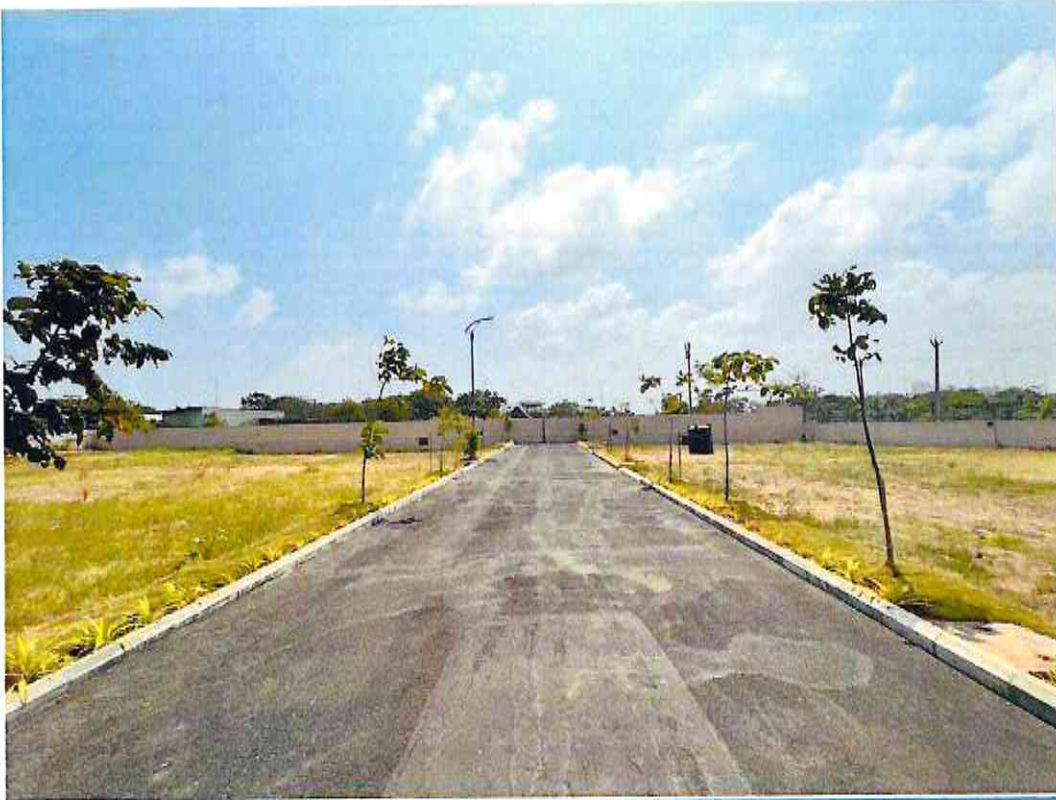
SITE PHOTO SHOLINGANALUR - II VILLAGE
