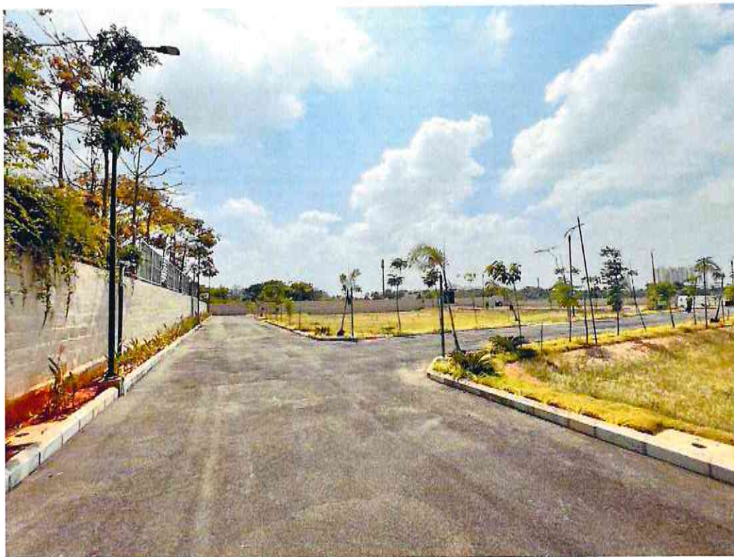
SITE PHOTO SHOLINGANALUR - II VILLAGE
