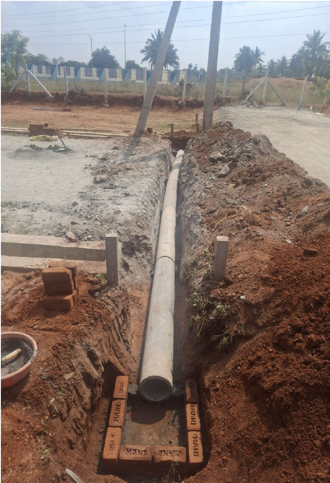
Photo Graph of the Mentioned Location During Construction Stage
